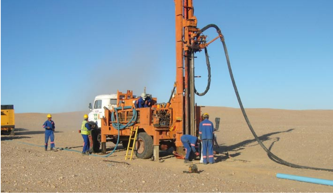
RC Drilling at Gawib West, Namibia – June 2007
